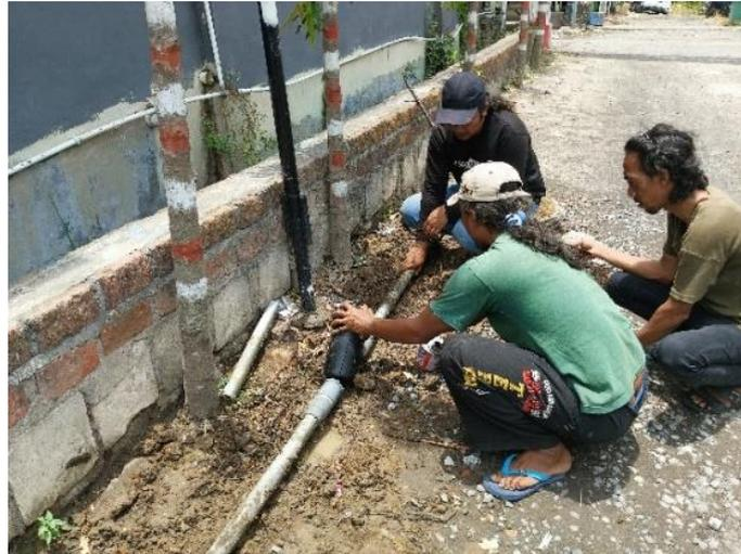
**Gambar 1: Pemasangan Sreen Filter**
